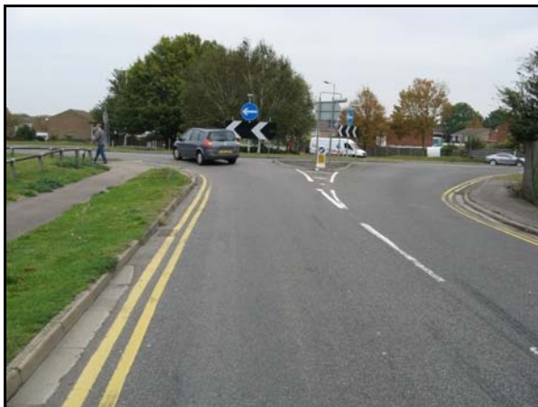
York Way approach, with insufficient space to allow widening to 2 lane approach
