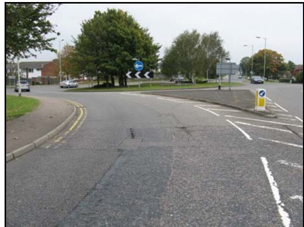
Old North Rd North approach to be widened to 2 lanes on the approach
