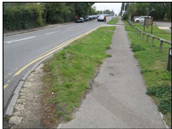
York Way approach, with double yellow lines to be extended to remove on street parking close to the roundabout
